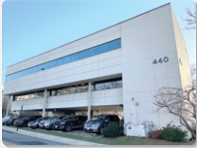
Starux, Inc. Headquarters in New Jersey
